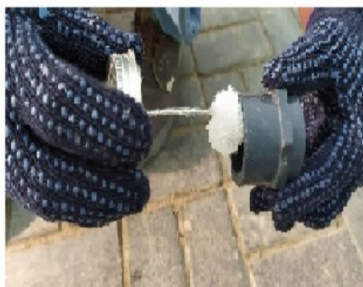
INSTALLATION OF PVC FITTINGS
