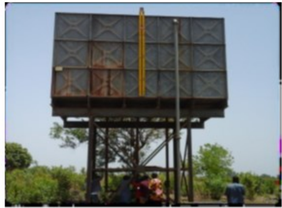
Leaking reservoir
