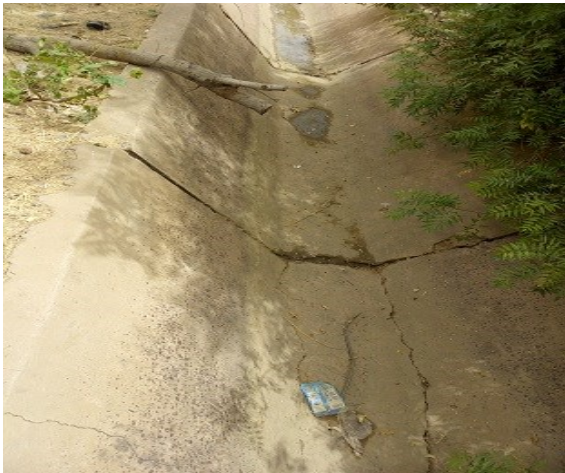
Broken canal structures
