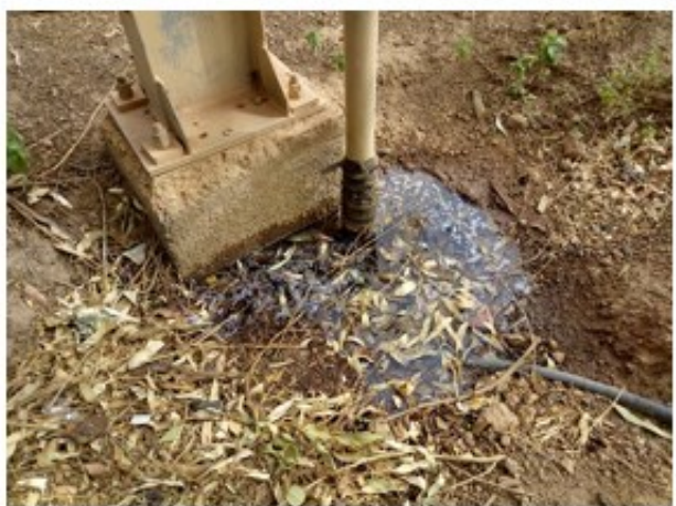
Leaking pipe
