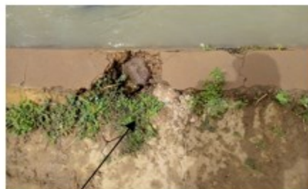
Cracks on the main canal
