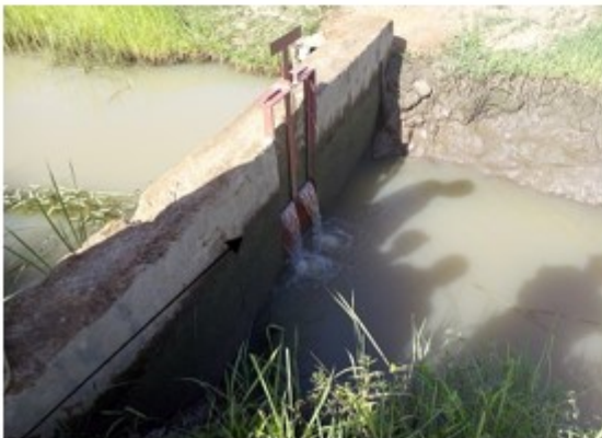
Leaking gate
