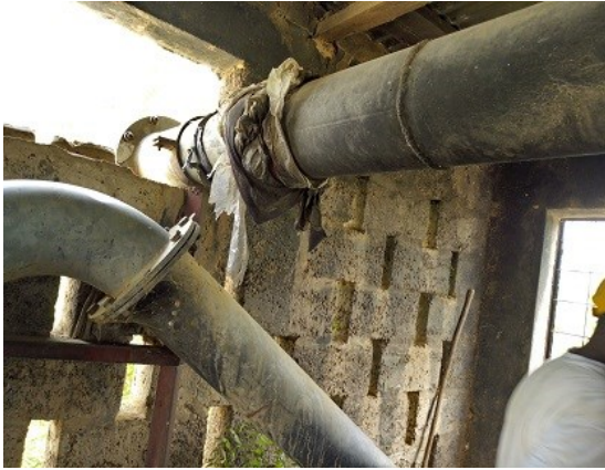
The main pipe due to leakage
