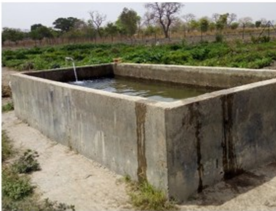
Leaking reservoir
