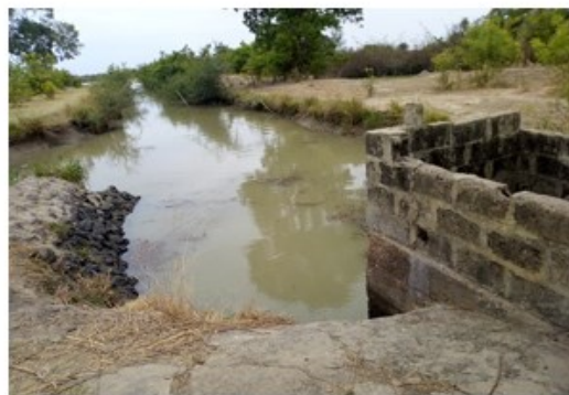
Eroded main canal from the river
