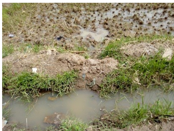
Sand-filled drainage canal
