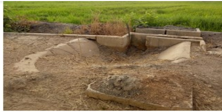
Distribution box filled with sand
