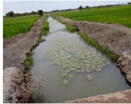
Eroded canal
