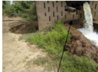
Eroded machine house
