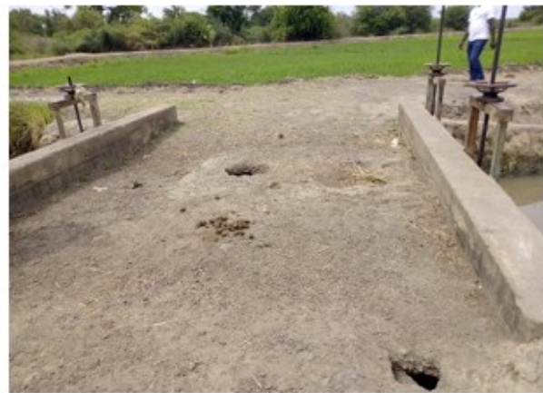
Potholes on the culvert
