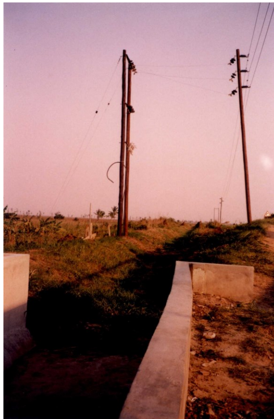
FIGURE 57. MAIN WATER DISTRIBUTION CHANNEL AND THE RESPECTIVE ELECTRICITY TP SUPPLY TO THE PUMPING STATION OF MUCELO SCHEME.
