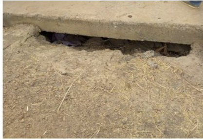
Collapsing culvert
