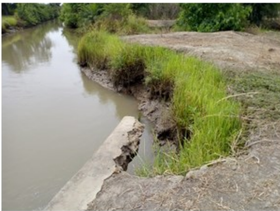
Erosion on the main canal
