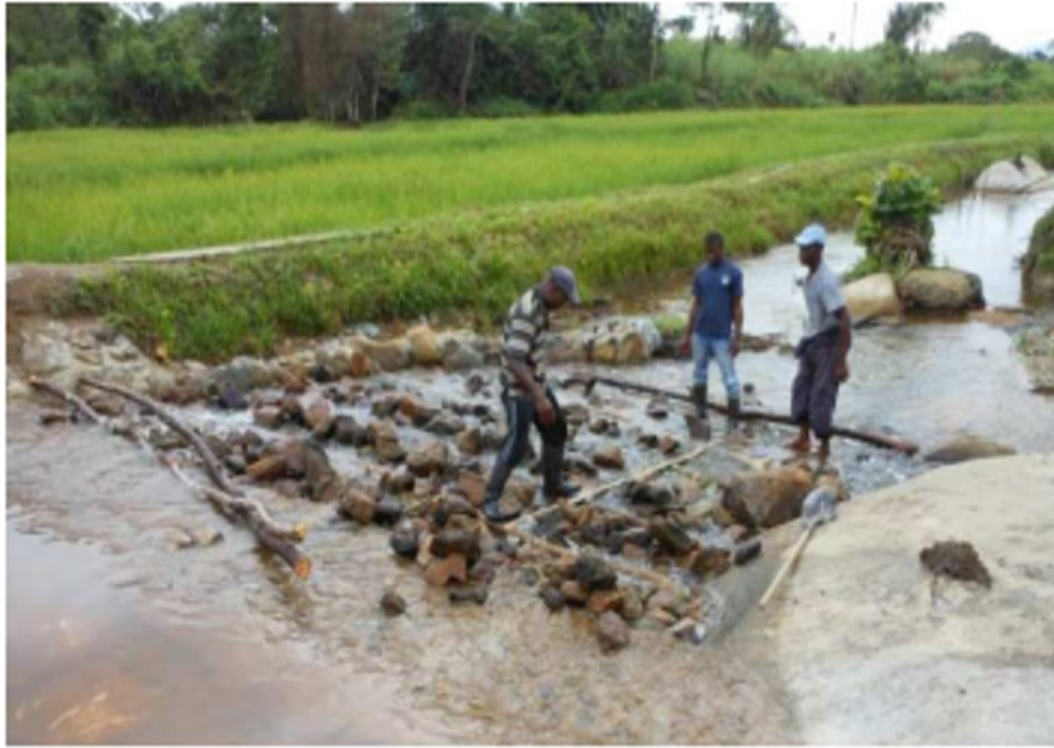
FIGURE 28. STONE-PAVED CHUTE FOR FLOODWATER DRAINAGE IN THE PROJECT AREA.
