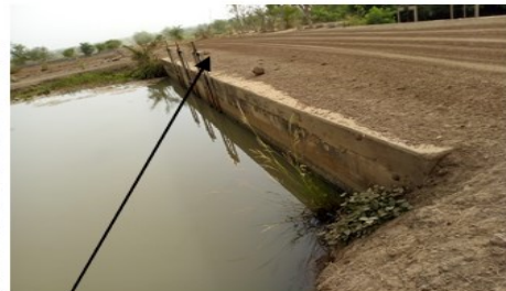
Leaking gates
