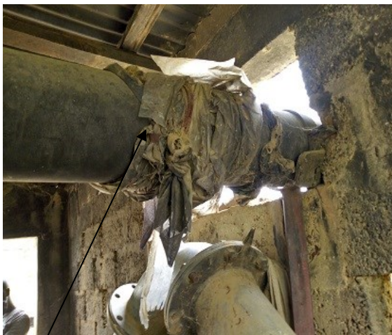
Management of leakages in main pipe
