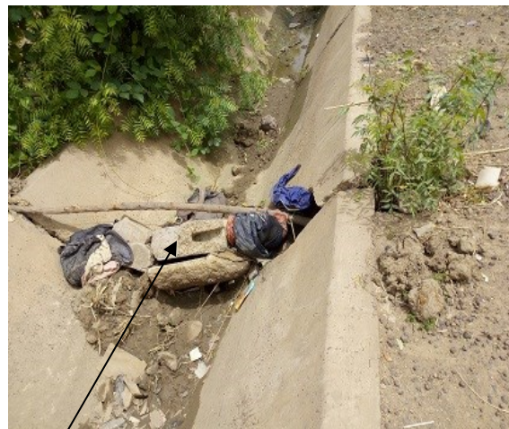
Attempt to block leakages in the canal
