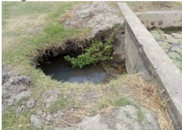
Collapsed culvert
