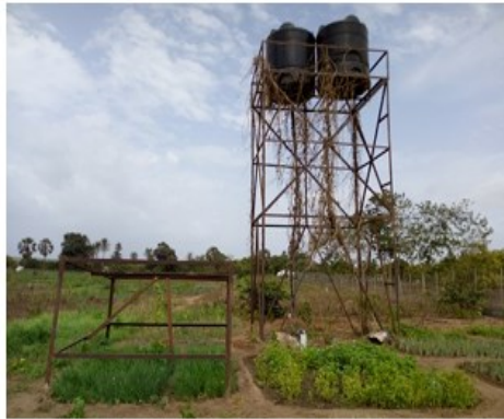
System not in use because of stolen panels
