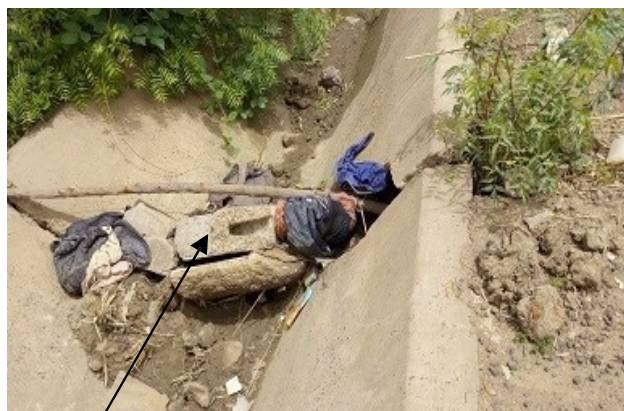
Attempt to block leakages in the canal
