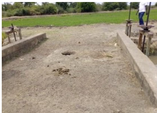
Potholes on the culvert
