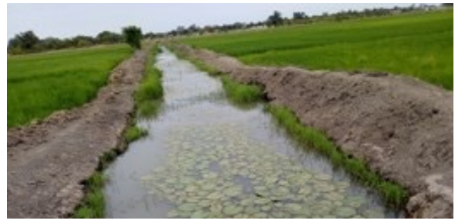
Eroded canal
