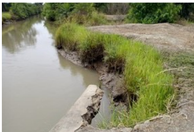
Erosion on the main canal
