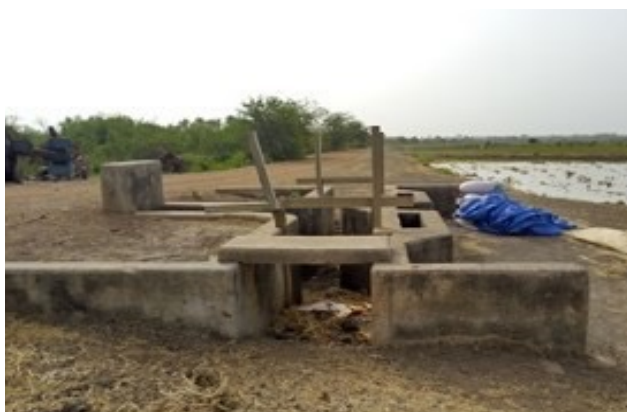
Old structure of the main distribution box
