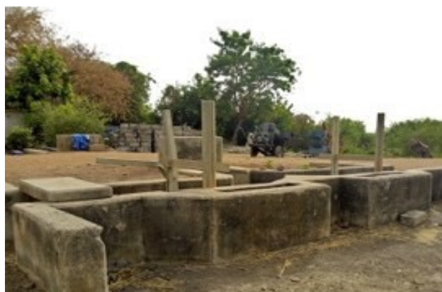
Distribution box filled with sand
