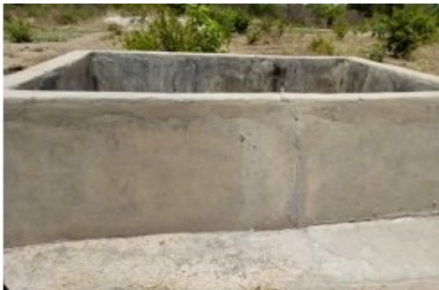
Cracks on the reservoir
