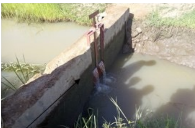
Leaking gate
