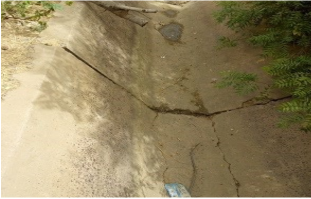
Broken canal structures
