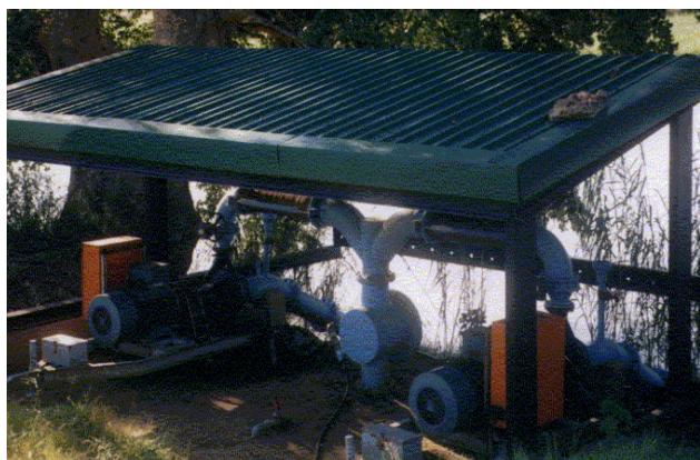
FIGURE 47. ELECTRIC PUMPING STATION OF DRIP IRRIGATION IN THE VEGETABLE PRODUCTION SYSTEM, INCOMATI RIVER, MOAMBA DISTRICT, MAPUTO PROVINCE.
