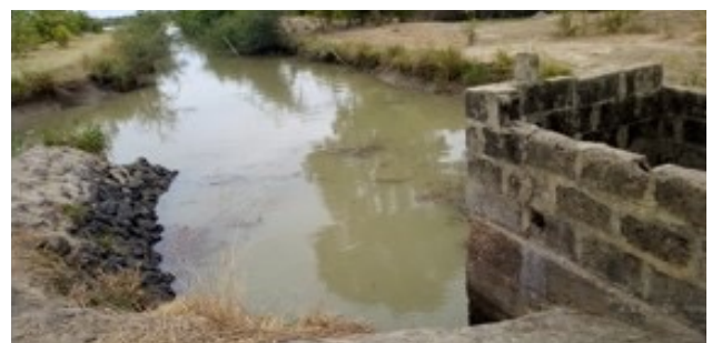
Eroded main canal from the river
