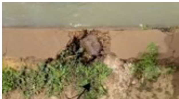
Cracks on the main canal
