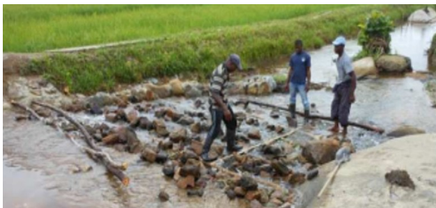
FIGURE 28. STONE-PAVED CHUTE FOR FLOODWATER DRAINAGE IN THE PROJECT AREA.
