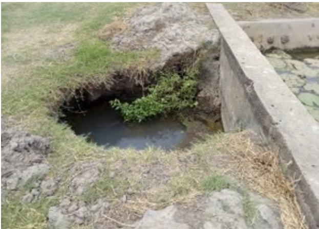
Collapsed culvert
