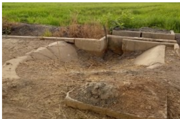
Distribution box filled with sand
