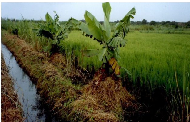
FIGURE 52. COMBINED TERTIARY IRRIGATION CHANNEL, DRAINAGE DITCH, AND CONSERVATION BANK (DINA, 1991).
