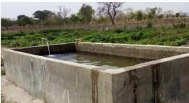
Leaking reservoir
