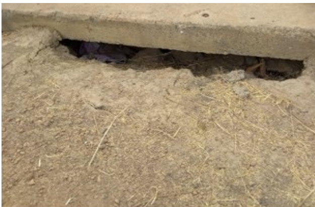
Collapsing culvert
