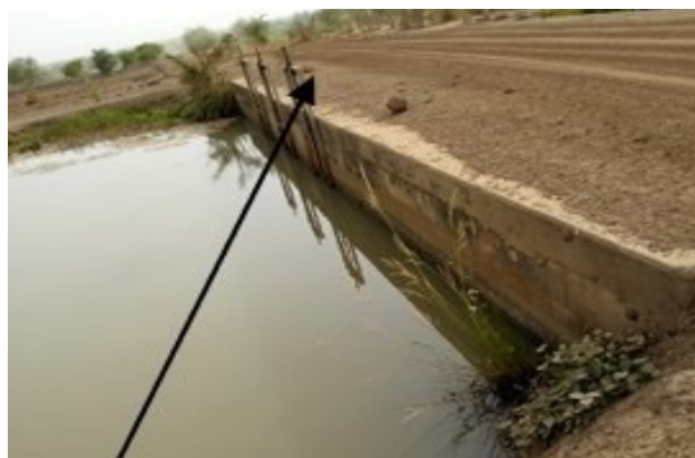
Leaking gates
