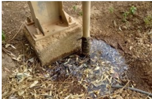
Leaking pipe
