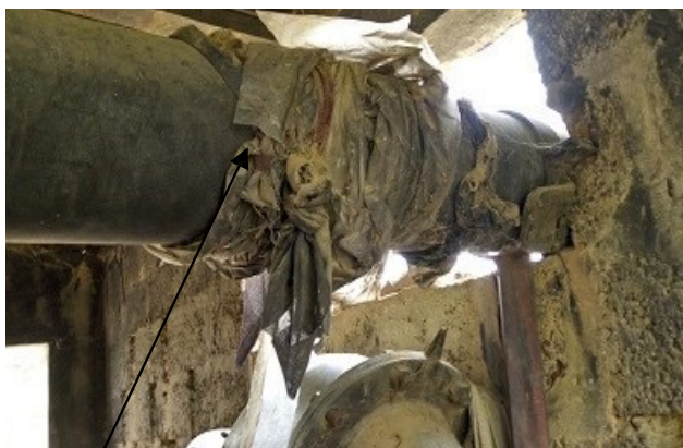
Management of leakages in main pipe
